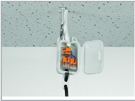
Pendant light connection in a suspended ceiling
