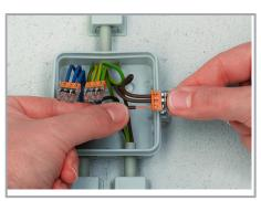
Termination: Insert the stripped solid conductor until it hits the backstop.
